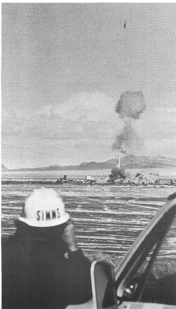
BLAST of Davis gun is viewed through binoculars by Bob Simms (1173) from safety area. Dark object above the gun is the 1830-lb. reaction mass which traveled over 4000 feet into the air and several hundred yards away from the test area.
